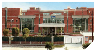
India Factory SMC Pneumatics (India) Pvt. Ltd. Total land area : 87,154 m 2 Total floor area : 43,939 m 2
