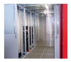
Cold-aisle containment in the data centre of Vitos Haina gem. GmbH reliably prevents hot and cold air mixing.
