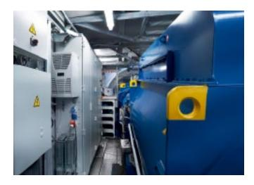
Converters in the nacelle are securely accommodated in TS 8 enclosures from Rittal. These enclosures are also spring-mounted on rubber bearings and steel beams at the top and the bottom due to the constant movements and vibrations.
