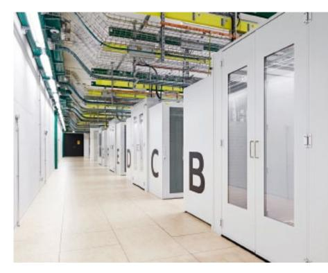
On completion of all four modules, the data centre will have 600 racks. With a good 25,000 U, it can accommodate around 6,000 servers and network components.
