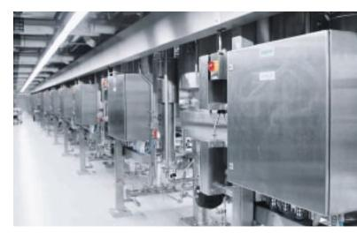
200 completely connection-ready stainless steel enclosures from Festo for the biotech factory's 80 batch containers and bioreactors with some 5,000 valve functions approximately.
