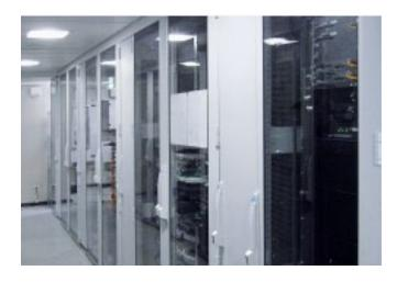
To stop it getting too warm in the narrow confines of the computer rooms on the luxury liner, the operator decided to air-condition the server racks directly using liquid cooling packages from Rittal.
