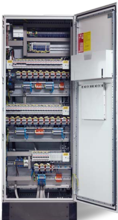
Works photo, WAGO
